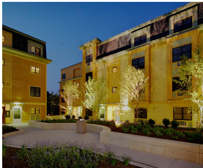
Intensive green roofs (12" to 3'-4' deep plant beds, engineered or conventional soil mix) allow a wider range of ornamental planting for attractive, useable rooftop spaces. (Source: Stantec)
