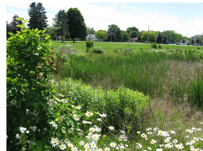
The existing bioretention pond, near Lakeway Drive, provides water quality volume sufficient to compensate for two remote campus improvements, where design of a conforming SMP was not practical.
