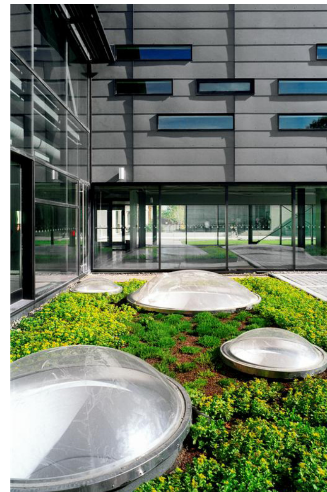
Extensive green roofs (6"-12" deep engineered soil mix, planted with sedums and ground covers) offer many environmental benefits, such as absorption of the storm water, insulation for the roof structure, and wildlife habitat. (Source: Stantec)
