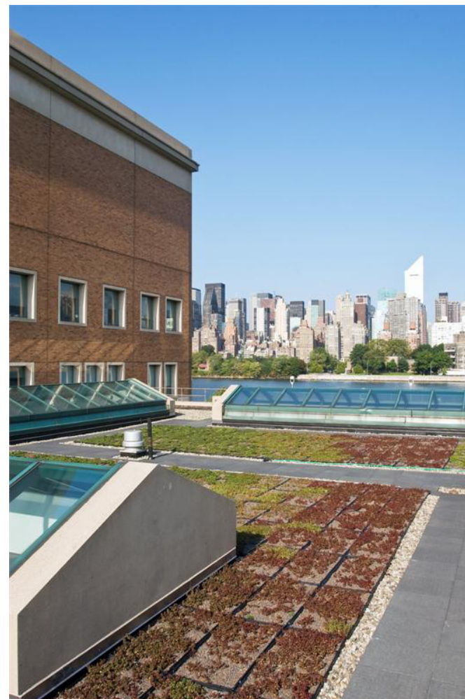
Extensive green roofs (6"-12" deep engineered soil mix, planted with sedums and ground covers) offer many environmental benefits, such as absorption of the storm water, insulation for the roof structure, and wildlife habitat. (Source: Stantec)
