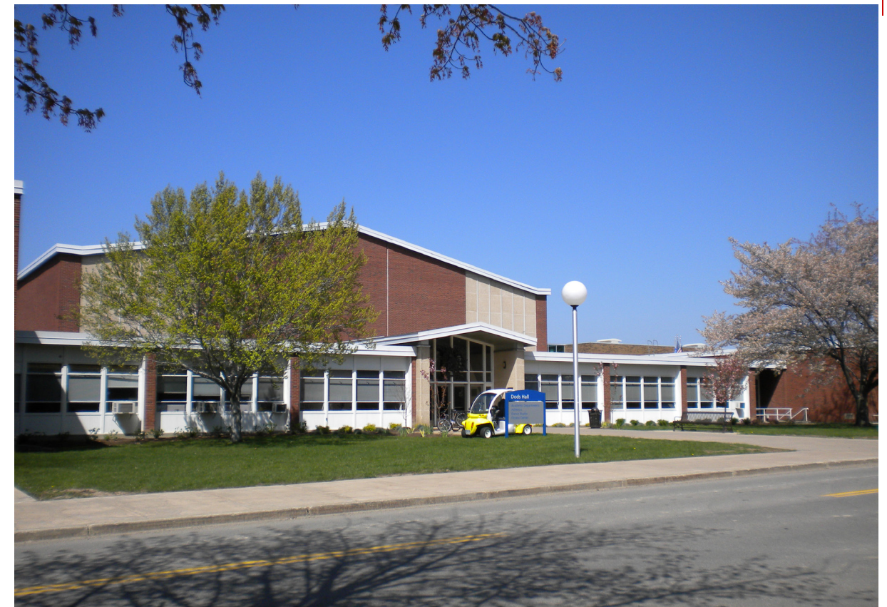
The existing Dods Hall entrance with the volume of the gym beyond. A new gymnasium structure also presents an opportunity to improve the appearance of the facility's main entrance.
