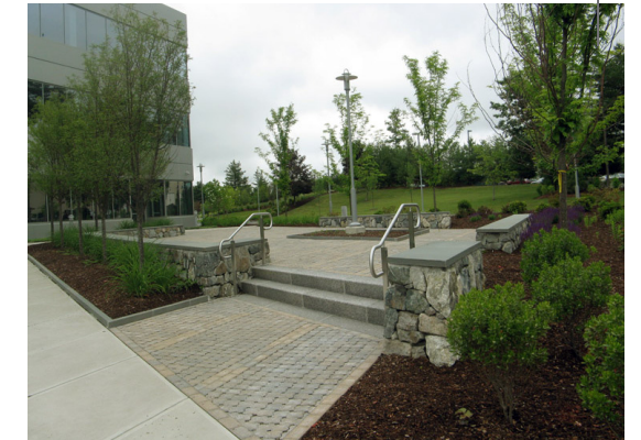
Permeable unit pavers are an attractive porous pavement choice for plazas and pedestrian areas.
